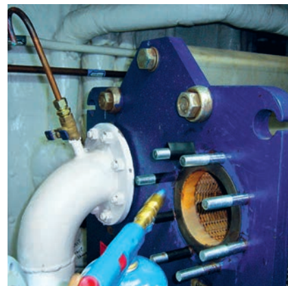
HEAT THE SHRINKING HOSE, SO THAT THE SHRINKING HOSE IS TIGHT AROUND THE BOLT
