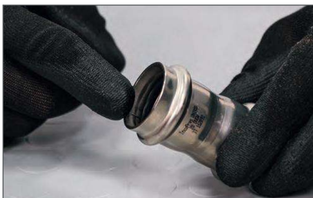
Controllo O-ring / Checking the sealing ring
